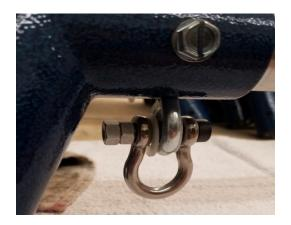
The Easy Glide Connection consists of a high strength shackle with screw pin, cable tie, two high strength polymer washers and a high strength polymer bushing. See the figures (*above*) for the assembly by itself and with it installed in the backbone eyebolt.
